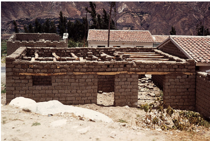
Adobe house under construction
