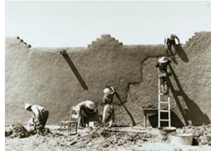
Adobe wall coating renewal
